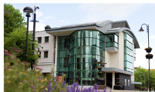
Palace Theatre, Town Centre
