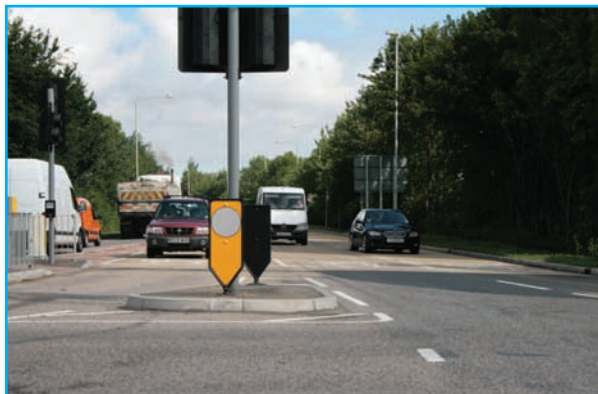
Keep left bollard, with rear face uncoloured
