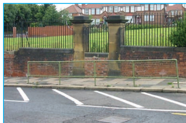
This guardrail has no function - the pedestrian route it was protecting has been closed - and can therefore be removed.
